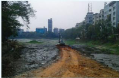
Lake Dewatering & Excavation
