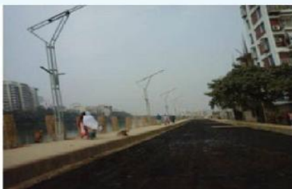
Road Construction & Street Lighting
