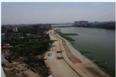
Lake Drive Road Construction at Badda
