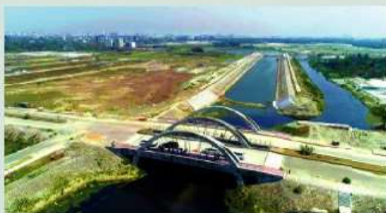
Progress work/ on going development work
