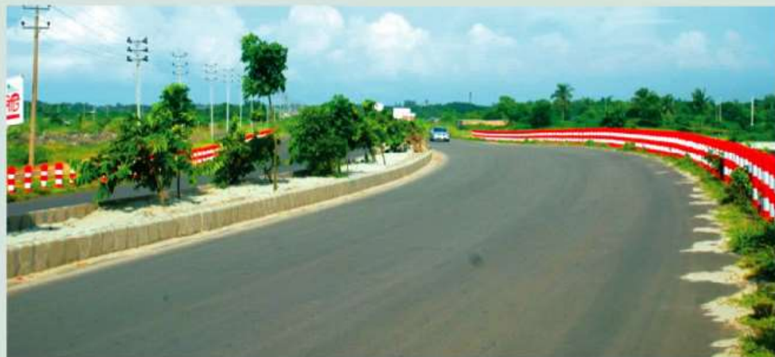
Fig: Ongoing development works in Purbachal New Town Project.
