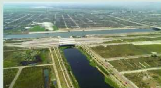
Progress work/ on going development work
